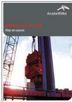
Installation of sheet piles GB, DE, FR
